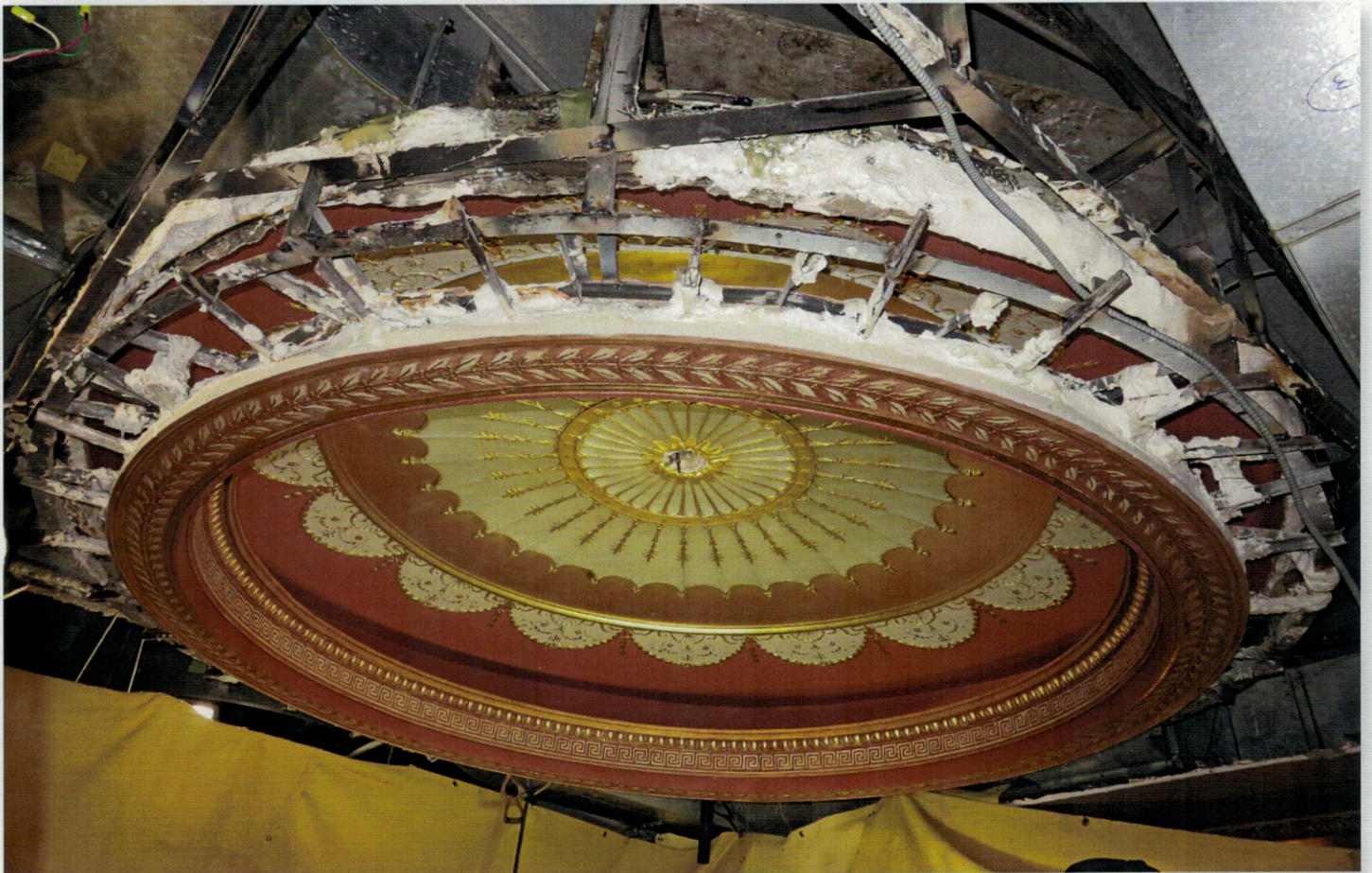
Plaster removal at the Lyric Theater
