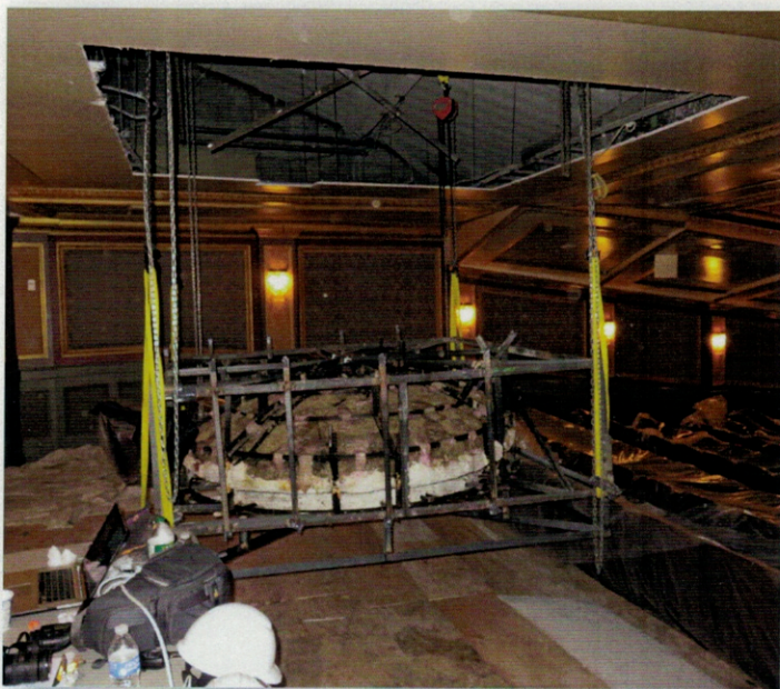
Plaster removal at the Lyric Theater
