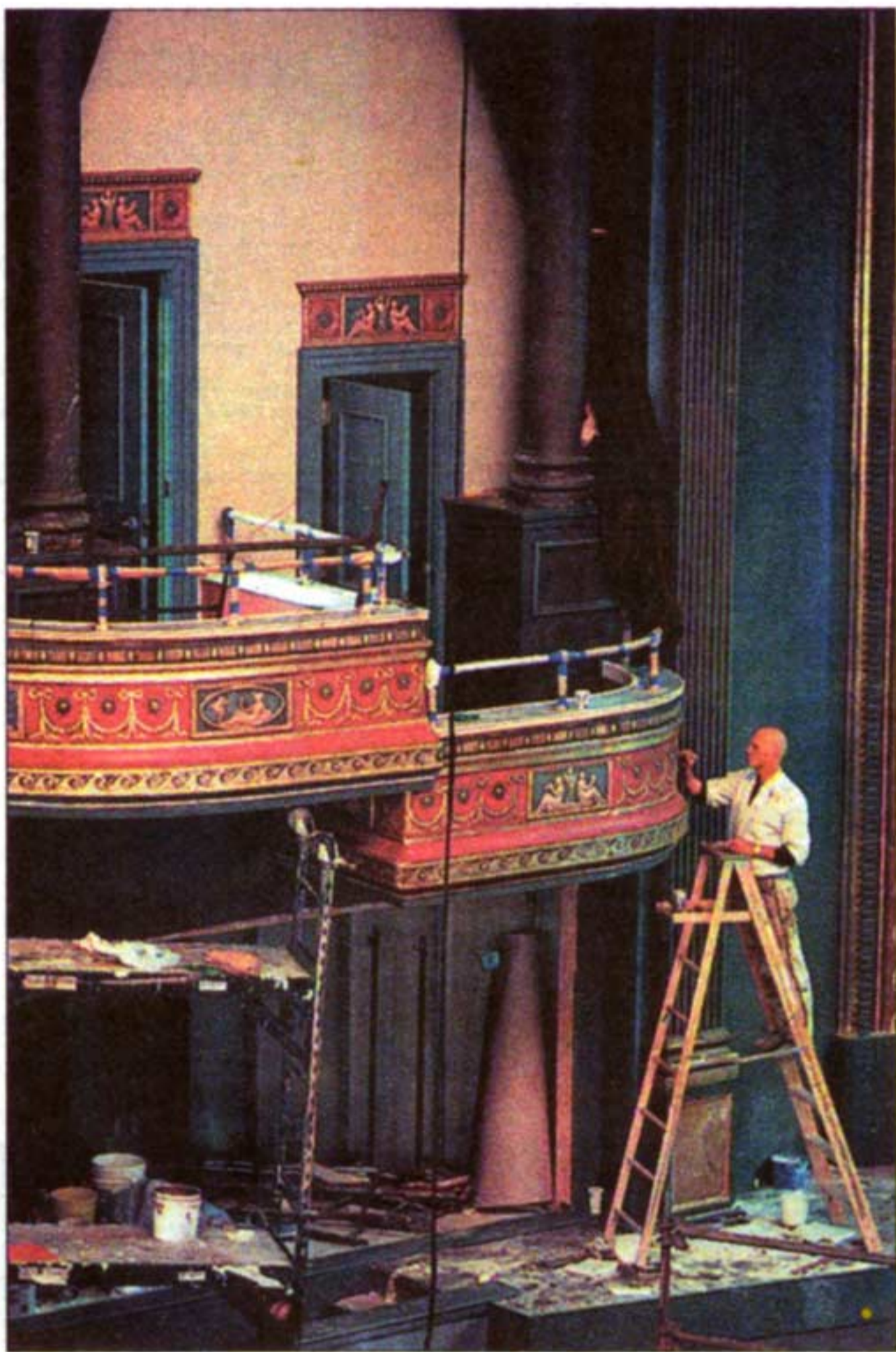
In November, side boxes were painted and gilded, left, and the Ford sign went up on 42nd Street, right. This month, "Ragtime" production crews moved into high gear in the finished 1,821-seat auditorium, below.
