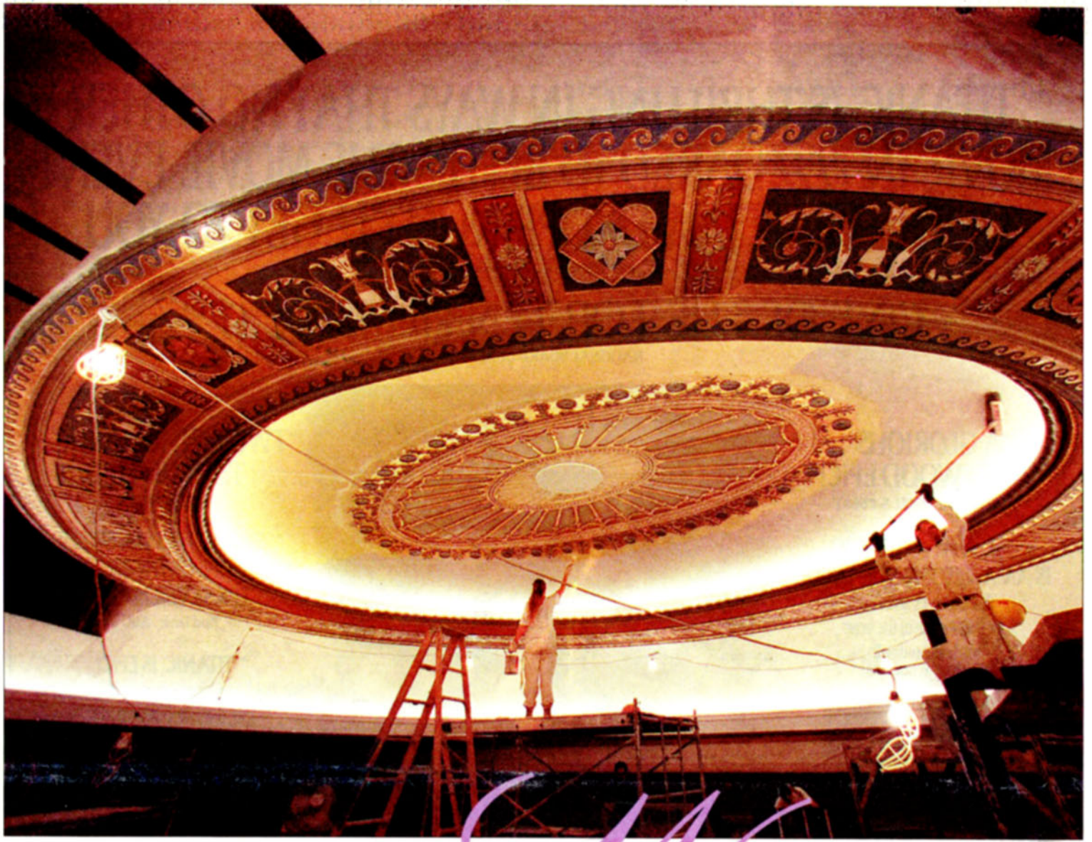
In April, only steel beams and girders framed the future orchestra section, below, where a worker cured just-poured concrete. In September, painters worked on the theater's ornate ceiling dome, which was salvaged from the Apollo and installed directly over the orchestra.
