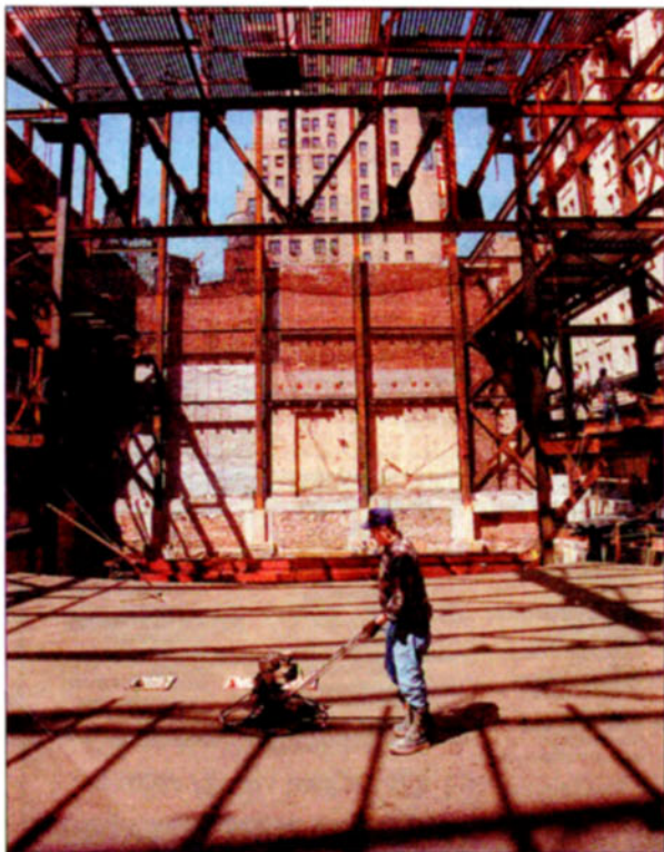
In April, only steel beams and girders framed the future orchestra section, below, where a worker cured just-poured concrete. In September, painters worked on the theater's ornate ceiling dome, which was salvaged from the Apollo and installed directly over the orchestra.
