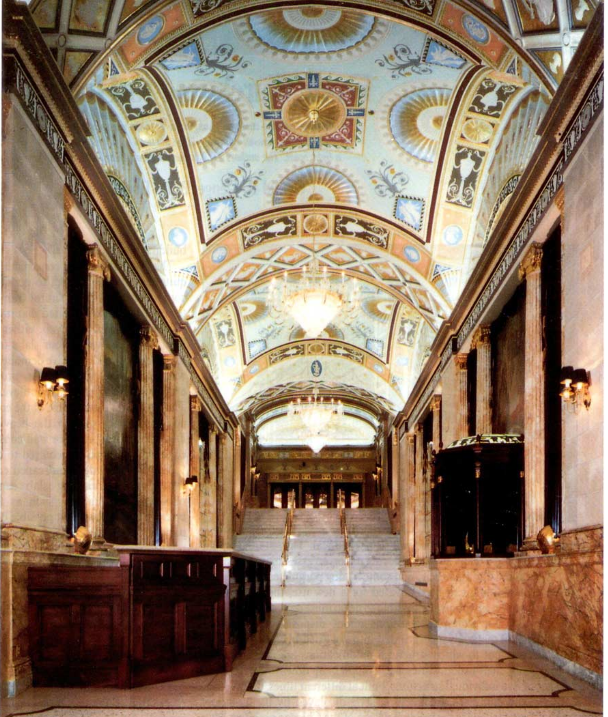
6 The luxurious 36-m link from Yonge Street, approaching the stairs over O'Keefe Lane and the entrance to the mezzanine lobby. Sprinkler heads are covered by brass plates to help them integrate with the ornate plasterwork, and individual heat and air induction units are concealed behind scagliola wall panels.
